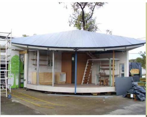
addition to the Vantage range of residential windows and doors. These innovative systems incorporate a thermal break to reduce the transfer of heat across the window frame, enabling better control over interior temperatures, to maximise efficiency and comfort. Architectural Windows Systems, in conjunction with AVS Windows and Doors, agreed to donate their knowledge, time and products to this unique project.
